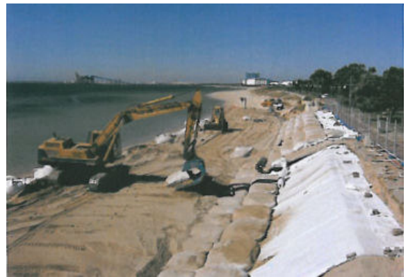
Figure 2 - Backstop wall under construction in Australia
